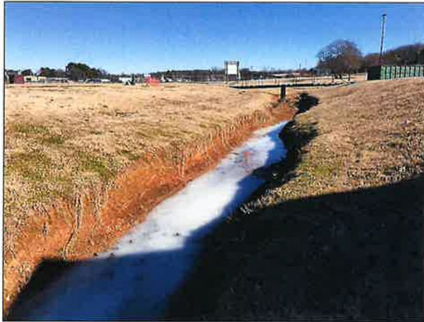
Illicit Discharge into Normal Branch
